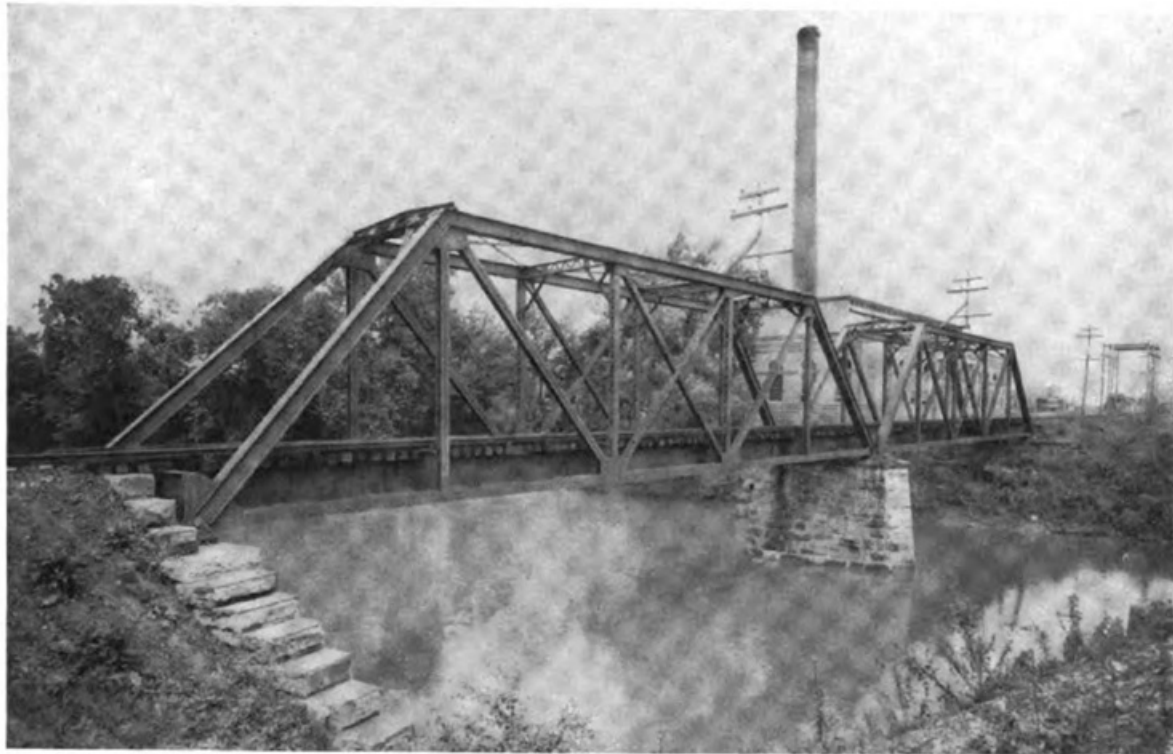
VIEW AT BIG WALNUT CREEK, SHOWING STANDARD BRIDGE CONSTRUCTION. POWER HOUSE IN BACKGROUND—SCIOTO VALLEY
