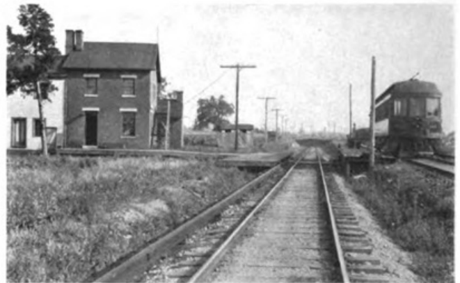
OBETZ JUNCTION, THE JUNCTION POINT OF LANCASTER AND CHILLICOTHE DIVISIONS. THE PASSENGER STATION PLATFORM EXTENDS OVER THIRD RAIL—SCIOTO VALLEY
