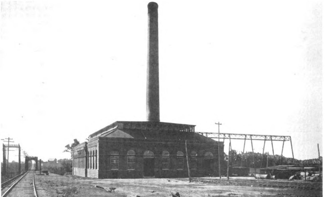
EXTERIOR POWER STATION, SCIOTO VALLEY
