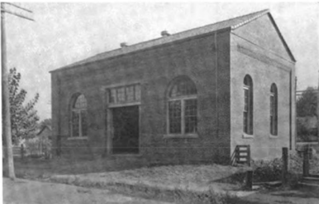
SUB-STATION BUILDING, SCIOTO VALLEY
