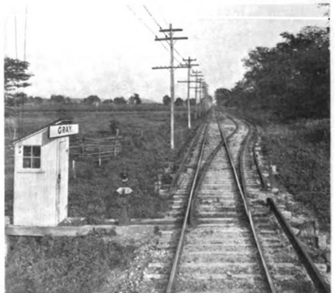
STANDARD TURNOUT, SHOWING SWITCH STAND, TELEPHONE BOOTH AND THIRD-RAIL CONSTRUCTION AND CONNECTIONS, SCIOTO VALLEY
